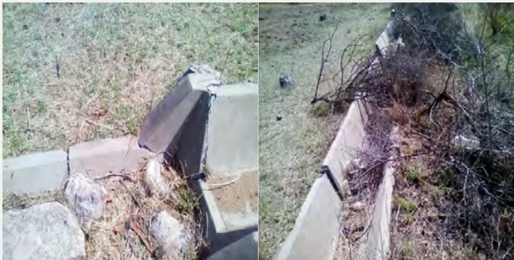
Condition of infield canals at Sebasa Irrigation Scheme (Source: International Fund for Agricultural Development no date)
